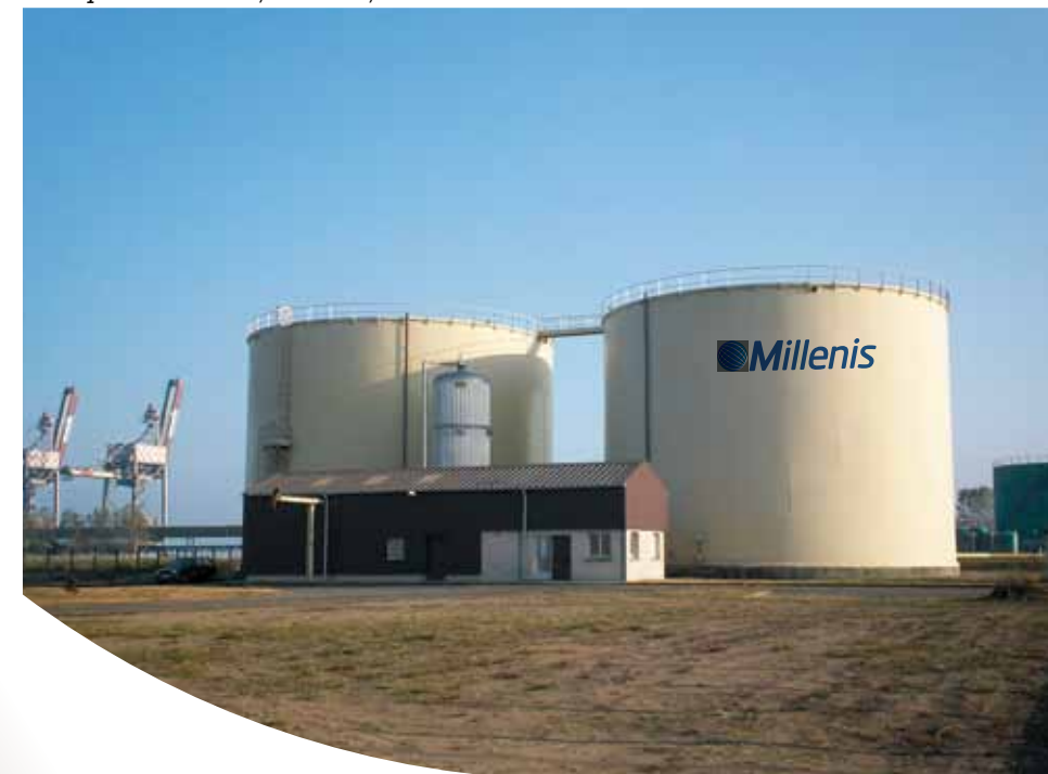
Liquids terminal, Montoir, France
